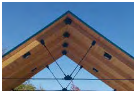
Rod and clevis ties
