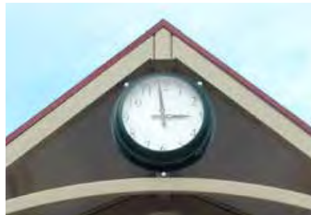
Clock and curved tie beam
