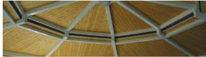
Interior view of vented roof option
