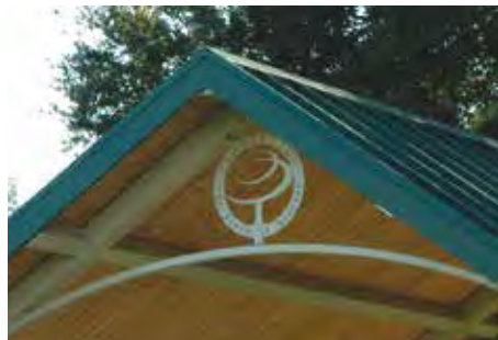
Curved tie beam with laser-cut medallion
